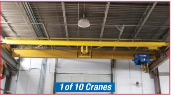
LOAD LIFTER 5 TON, 30' X 90' CRANE
